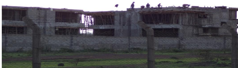
Plate 6: Construction going on 5 metres from Wilson Airport along Runway 07 Source: Author (2014)
